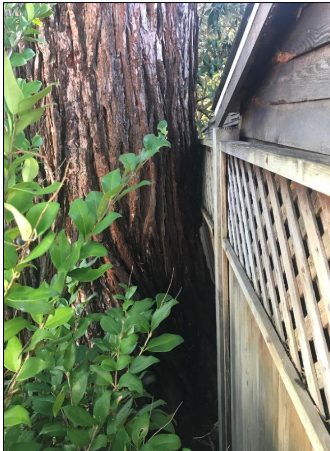
Figure 4. Trunk conflict with fence and structure on 126 Suffield Ave. property.
