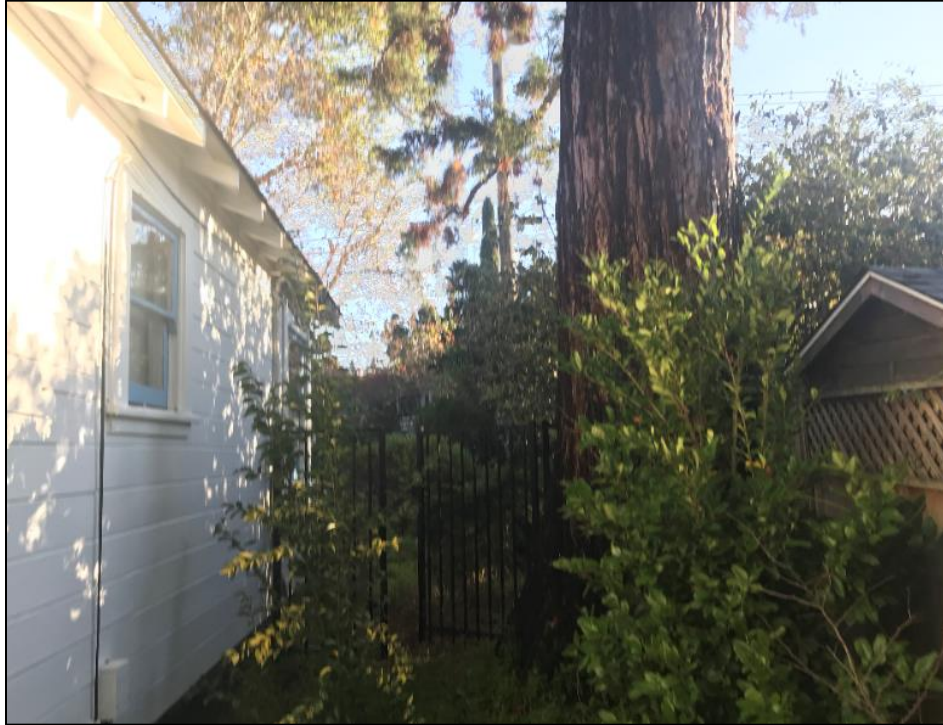
Figure 5. View of the trunk proximity to the home at 104 Suffield Ave.
