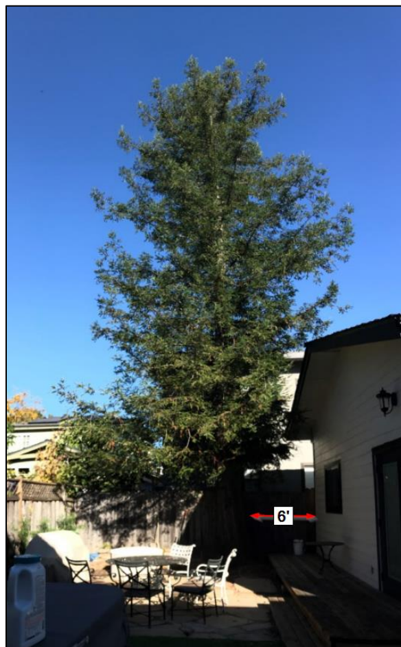
Figure 1. Subject tree as viewed from the Nielson backyard. Note the main trunk stands 6 feet from the foundation of the guest house (right).
