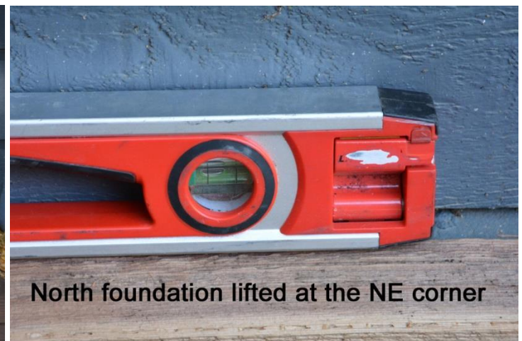
Figure 6a & b – The east and north foundation sections are lifted toward the NE corner and subject oak tree.
