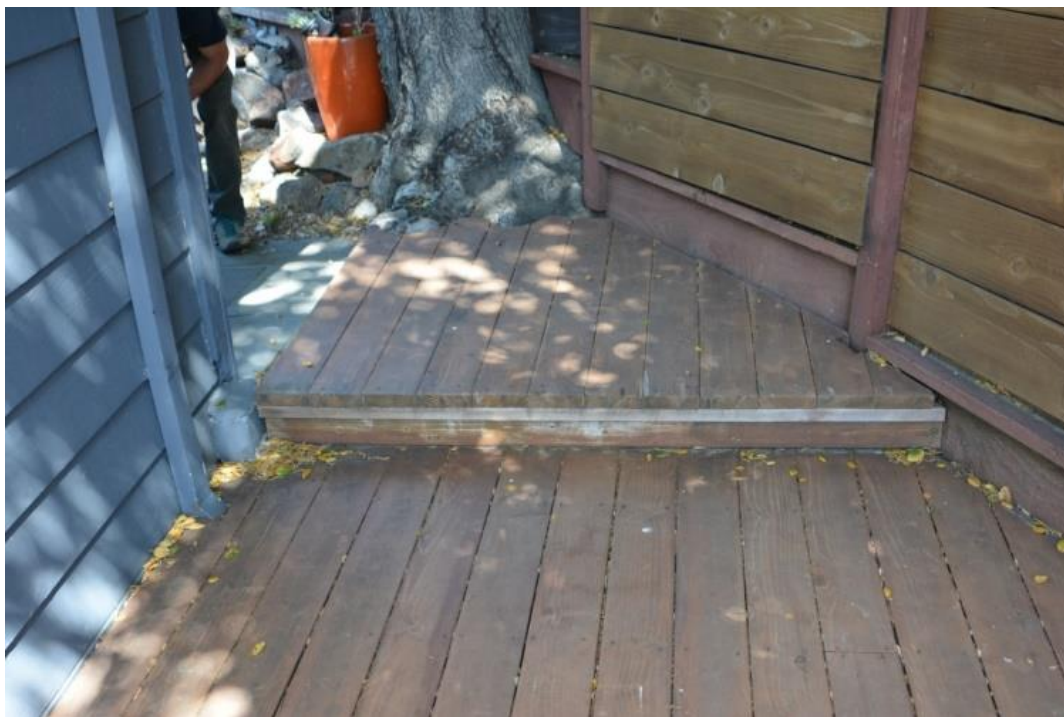
Figure 2 – The root system is limited by the house foundation and infrastructure.
