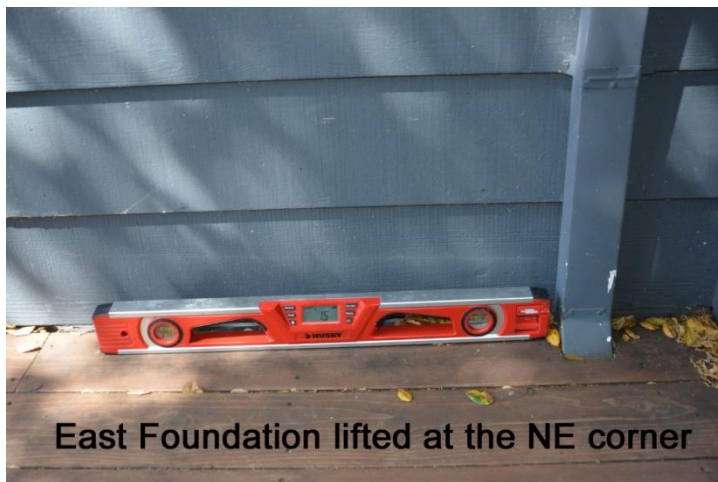
Figure 6a & b – The east and north foundation sections are lifted toward the NE corner and subject oak tree.
