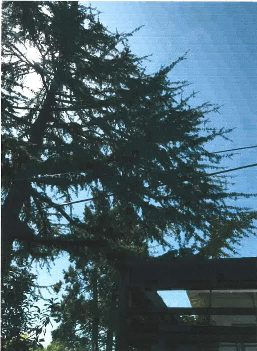
Figure 2. Proximity of the canopy to the home and roof.
