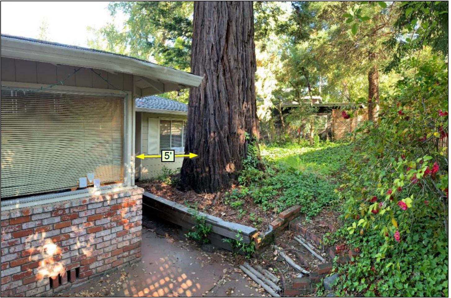
Figure 2. Proximity of the tree to the home and entryway
