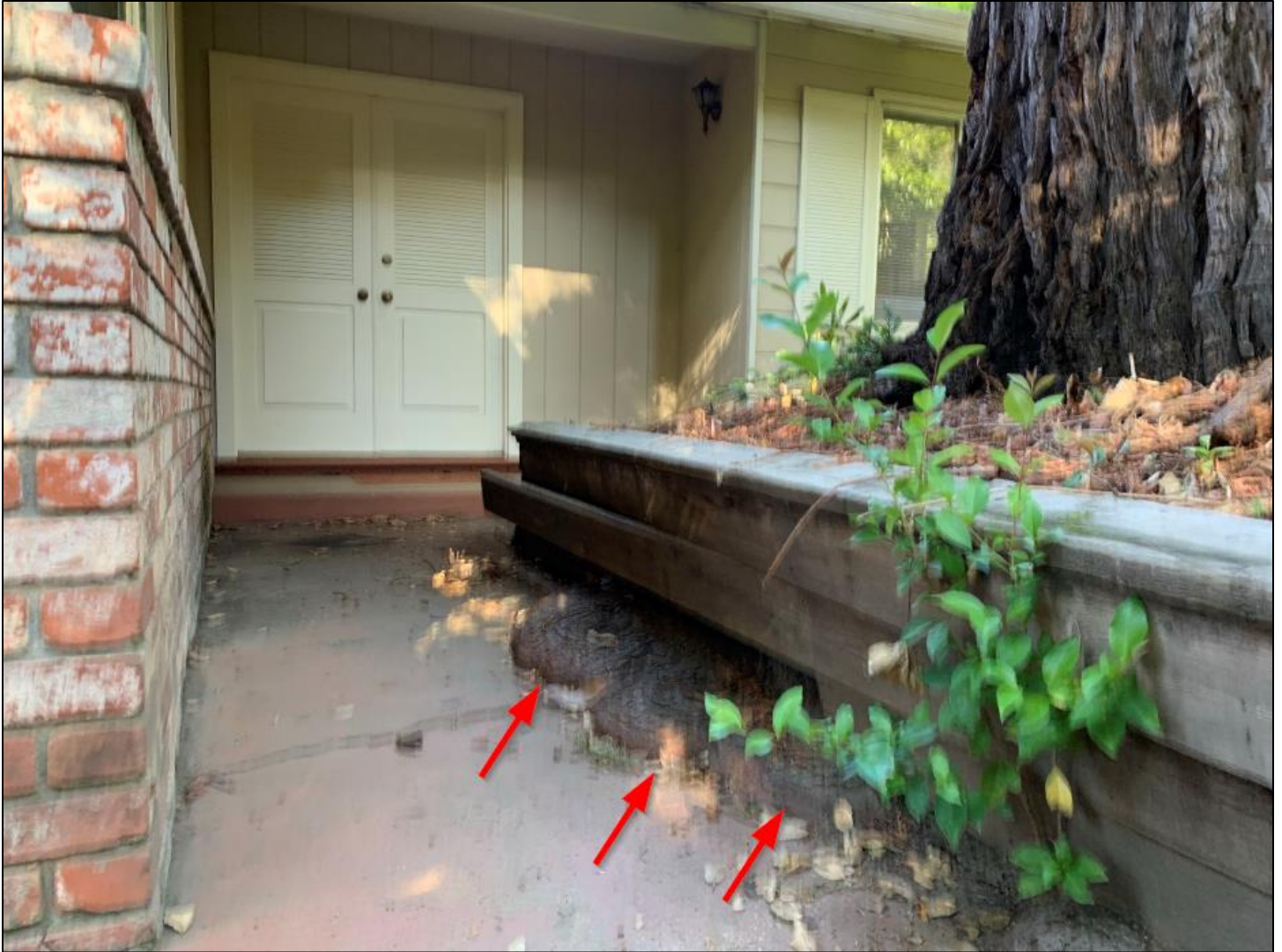
Figure 4. The shot is out of focus; however, the red arrows indicate root growth within three feet of the home.
